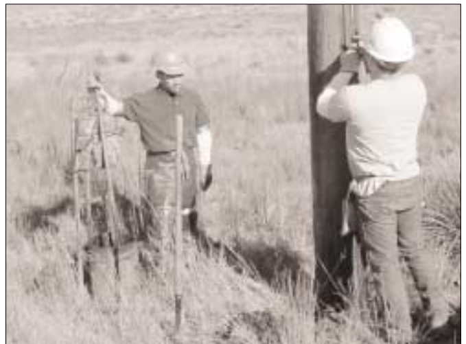
Technician sounds pole with hammer to check structure for voids.
