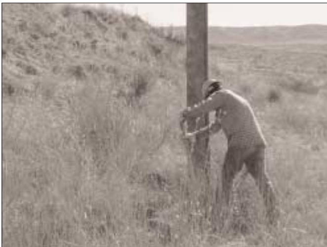
Worker digs 18-20 inches of soil away from the pole.
