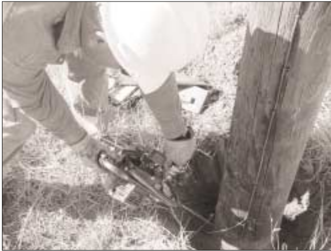
Technician drills a hole below the soil surface.
