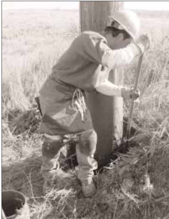
Wood preservative is applied to every pole after inspection.
