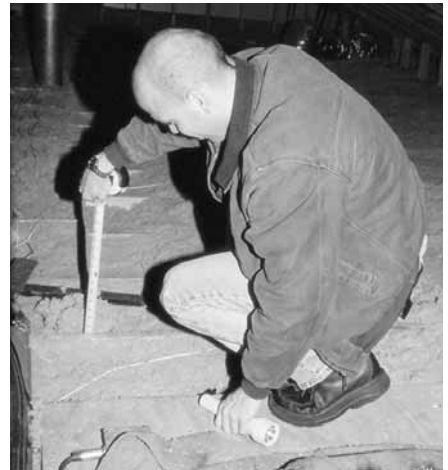
Installing attic insulation is an energy saver.
